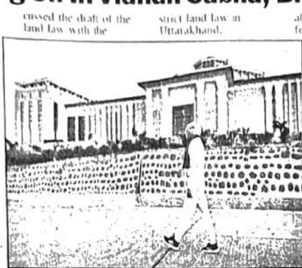
Chief Minister Pushkar Singh Dhami inspected the development works going on in Vidhan Sabha, Bhararisain on Thursday morning during his two-day Sansam tour.
